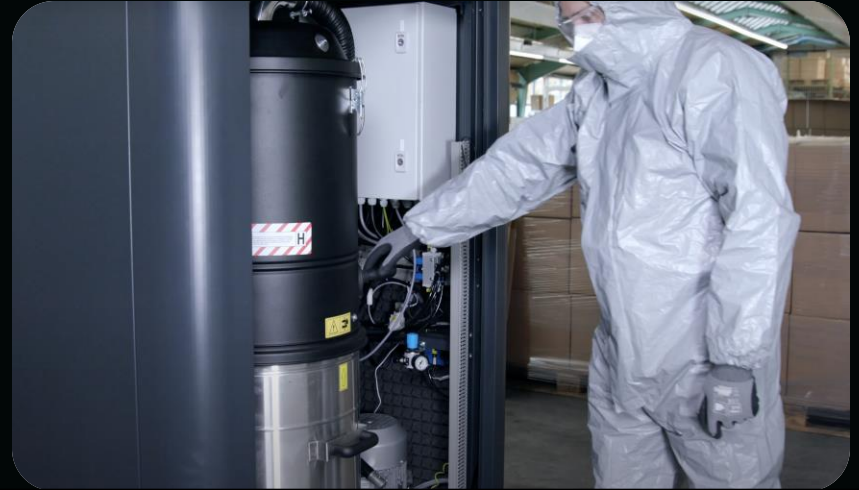
Easy access for maintenance
