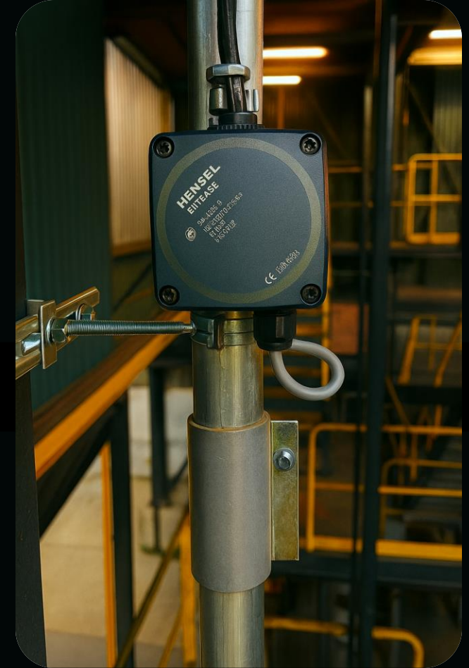
Electropneumatic valve
